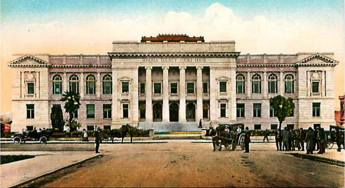
2419 - SONOMA COUNTY COURT HOUSE, SANTA ROSA, CALIFORNIA.
